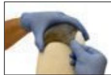
Position the tailored carbon fibre sections on those parts of the reinforcements that are to be strengthened, and at the same time pre-tension them in the fibre directions.
